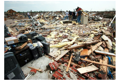
Office of SNC 2 after the 2011 Joplin tornado
